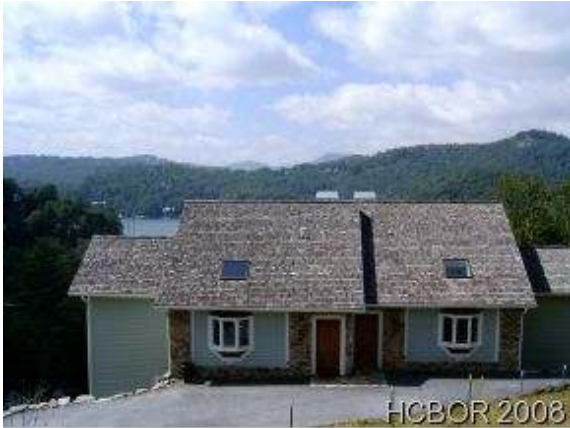
Front of building
